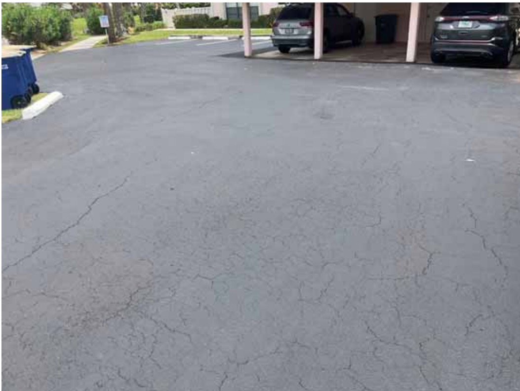
Pavement, Asphalt - Parking Area
