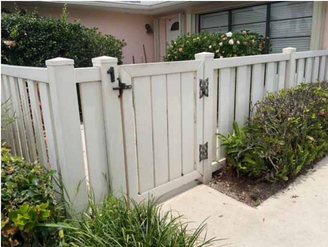
Bldg Courtyard Fence & Gate
