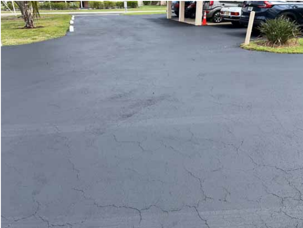
Pavement, Asphalt - Parking Area
