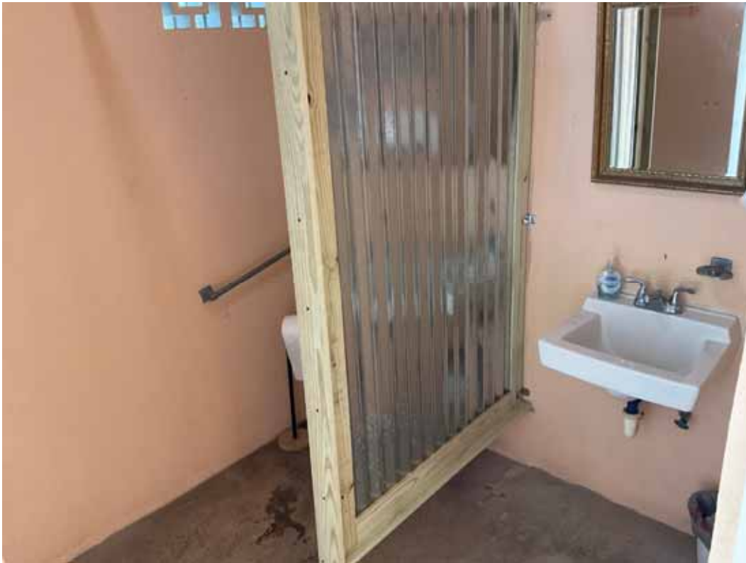
Pool Bldg Restroom, Women's
